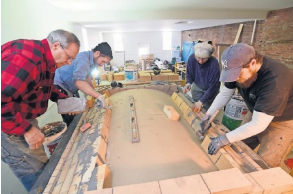
Workers install bricks on the dome of a bread oven Thursday as efforts continue to resurrect the bakery by the Old Labor Hall in Barre. From left are oven expert Dan Wing, of Corinth, master builder Jeremiah Church of Boreal Heat, Carolyn Shapiro, chairwoman of the bakery project, and Jamie Duggan from the State Division for Historic Preservation. JEB WALLACE-BRODEUR / STAFF PHOTO
